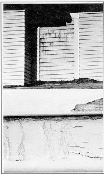
Figure 2. A streaked type of water soluble extractive discoloration can result from water wetting the back of one piece of siding and then running down on the front of the next piece.
